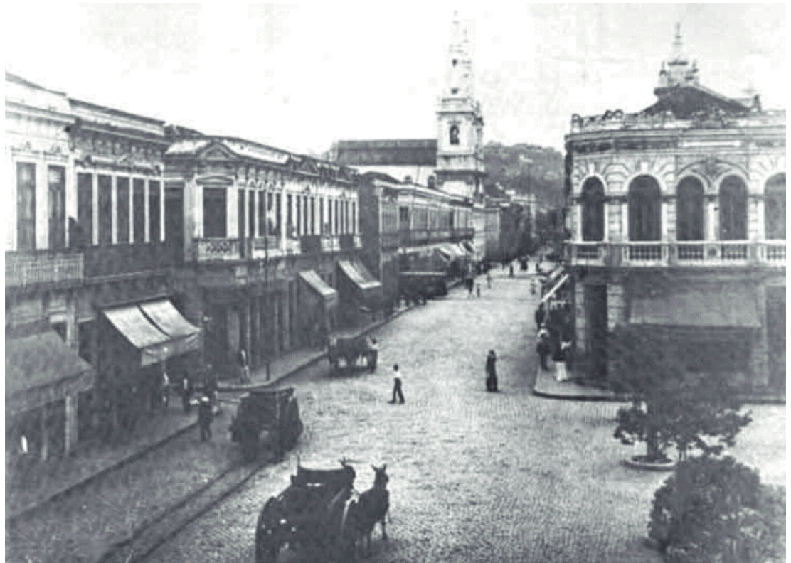
Figure 14: Sacramento Street and Largo de São Domingos after the construction works (1905).
