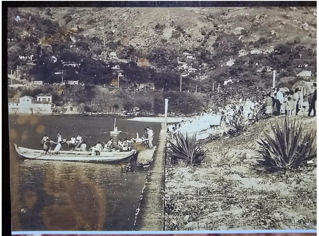
Figure 3: Workers disembark at Marambaia for bridge construction; Port House is visible in the background.
