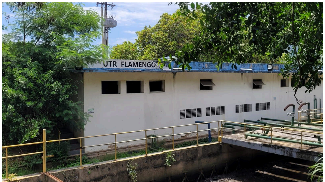
Figure 2: Photograph of UTR Flamengo. Source: Personal collection, January 2025.
